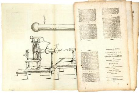
instrument-maker J. C. Gütle, responsible for installing the first lightning rod in that city. His machine demonstrates a method of generating static electricity from the rotation of a thin glass wheel, illustrated in detail in the folding engraved plate.
